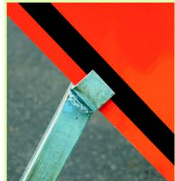
Sign clips hold bottom of rigid sign in place
