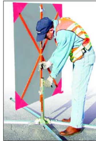
Rectangular signs need third vertical rib to secure to stand, and flex during wind gusts
