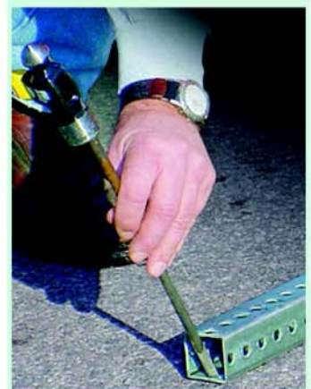
For extra stability, stakes can be placed through perforations in place of sandbags
